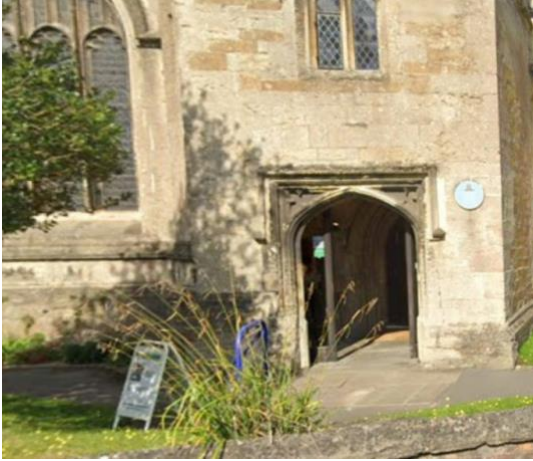
Level access door to the building which is wide enough for wheelchairs.
